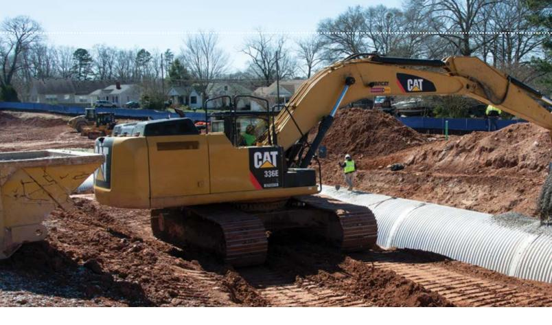
roughly 50,000 cubic yards of dirt, installing a 144-inch underground detention system approximately 600 feet in length, plus several other utilities that
